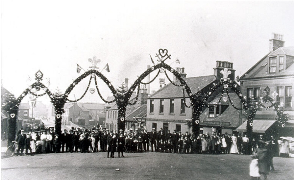
The 1908 Arch, the towns first 5 span arch
