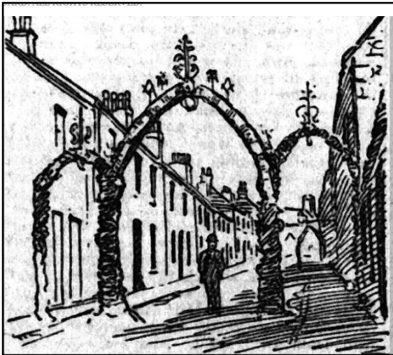
Figure 3 Sketch of Triple Span Gothic Arch in Cochrane Street from West Lothian Courier report 1901. There is also a small single span arch over the pavement on the right hand side of the image.
